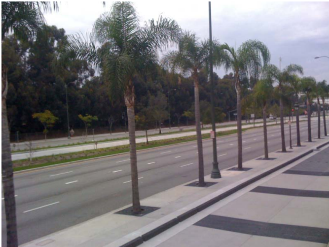
Photograph 3 – Santa Monica Boulevard Busway looking northeast
