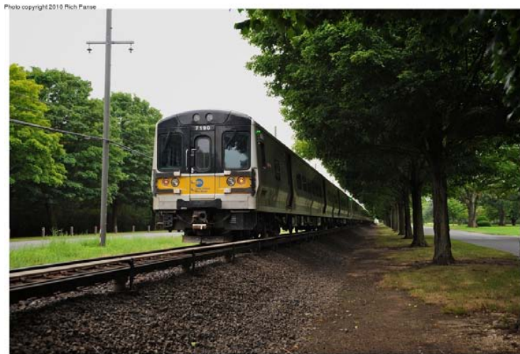
Photograph 2 – Long Island Railroad Third Rail
