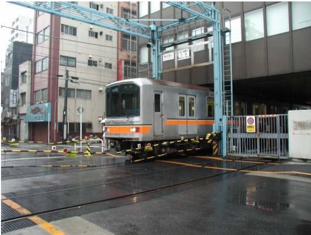
Photograph 4 – Third Rail Grade Crossing in Tokyo
